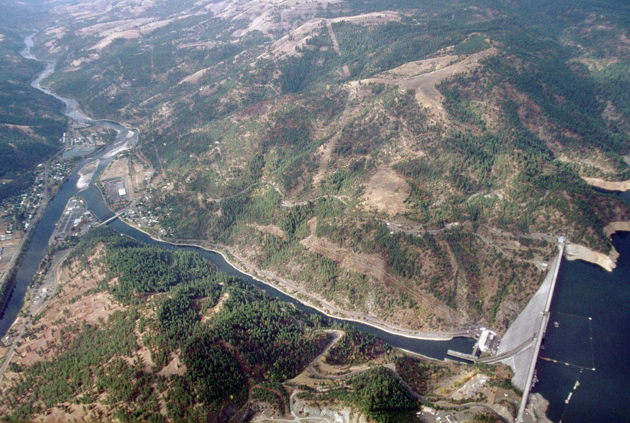
Dworshak Dam and Clearwater River view to the west.
